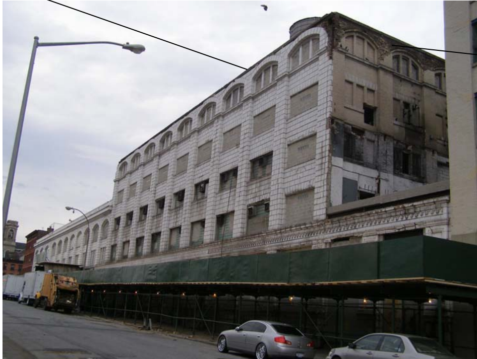
Photo 1 shows the entire Pacific St parapet lost due to collapse.
