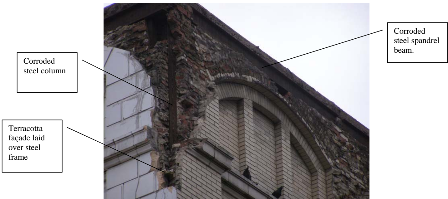
Photo 4 shows the close relationship between structural steel and ornamental façade
